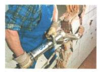
As a demolition tool, the DARDA HCS 6 **B** replaces the sledge hammer as a very efficient tool that will precisely break through brick walls up to 32 cm (12,6 inches) thirk
