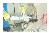
The HCS 6 J is able to crush concrete walls up to 15 cm (5,9 inches) thick (depending on compression strength of the concrete). A big advantage for breaking, separating walls, facade or reclamation concrete panels.
